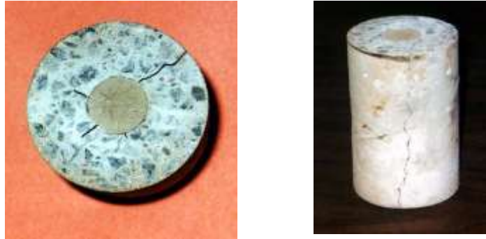
Figure 1 Thermal cracking due to transverse expansion of GFRP [5]
